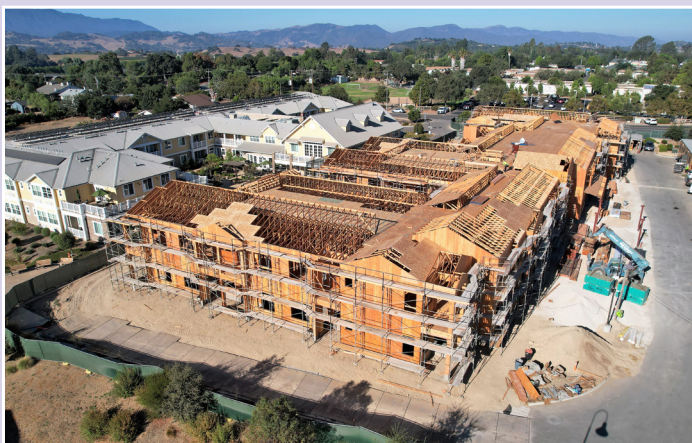
Photo provided by Sunseri Construction, Inc.
